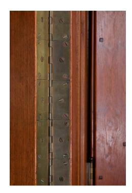
Built to take a licking and keep on ticking. Stacking butt hinges was a common practice for the Greenes. This stack helps support the substantial living room doors in the Thorsen house.
