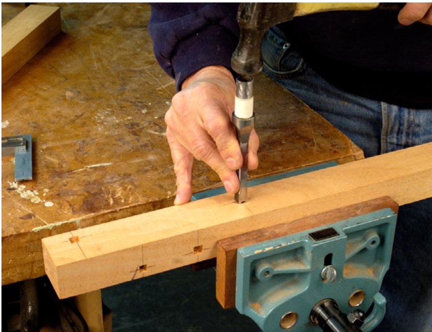
Driving home the point. The square chisel is placed back in position and hit with a hammer. After you reach the proper depth, use a small chisel to clean up the remaining waste.
